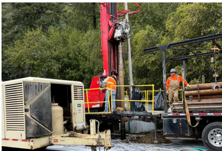
[Image description: Two men operating large machinery to install a well at Shelterwood.]
